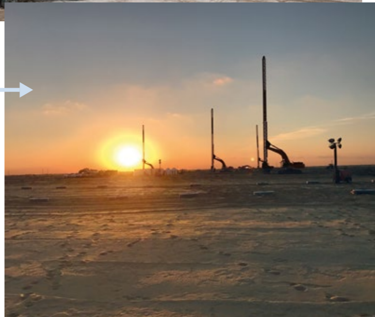
East Industrial Area - Free Trade Zone Port Said, Egypt
