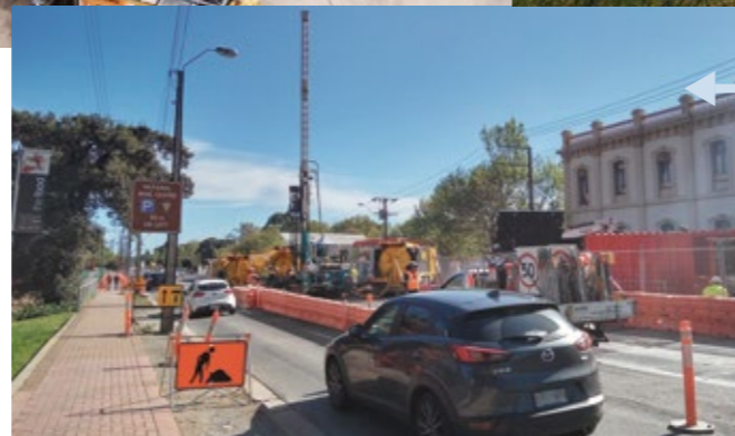
O-Bahn city access project Adelaide, Australia
