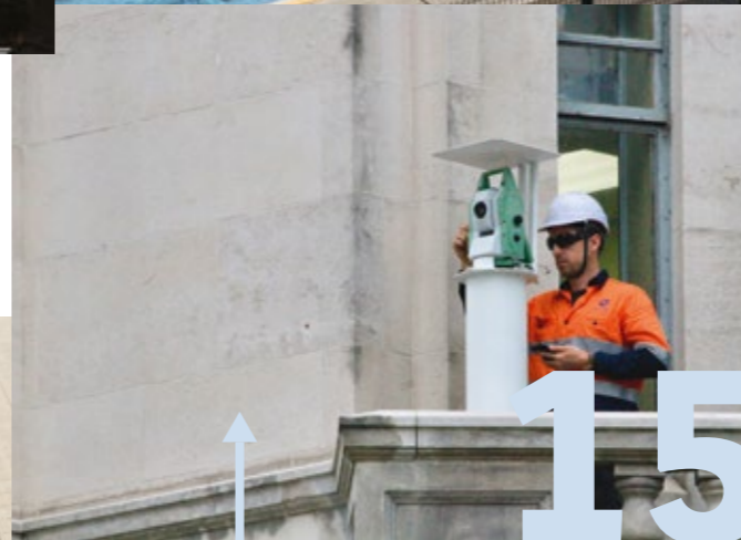
City Rail Link Auckland, New Zealand
