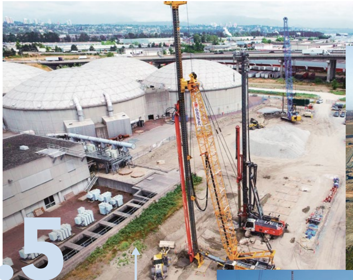
Annacis Island wastewater treatment plant Delta, British Columbia, Canada
