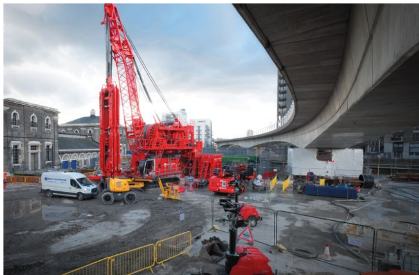
Thames Tideway Tunnel, United Kingdom
